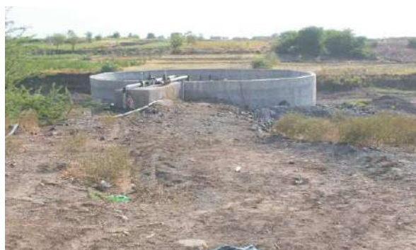
Percolation well for lift irrigation system
